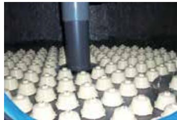
Nozzle Plate under drain system
